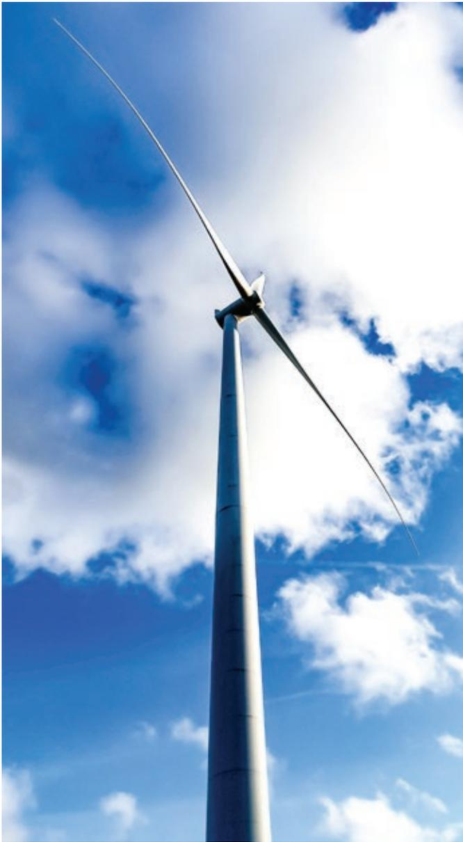
Wind turbines used for offshore applications are generally larger than onshore and are up to around 150m in diameter with a top blade tip height of around 180m (the height of the central hub around which the blades rotate is over 100m).
